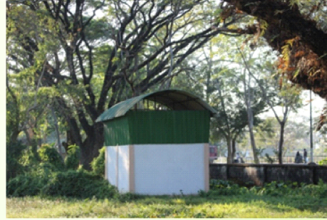
Incinerator in the GU Campus
